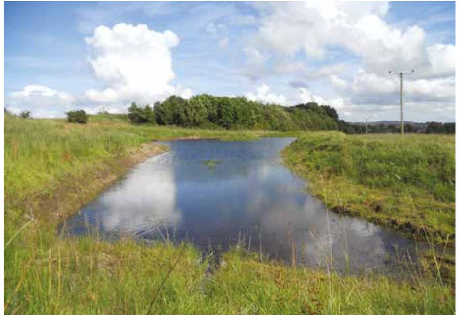
Figure 2.31. An offline storage pond in the Netherton Burn catchment, Northumberland: The pond has been designed in such a way as to offer additional water storage in times of high flow. The pond is supported by a series of sediment traps on the inflow points (© Tweed Forum).
