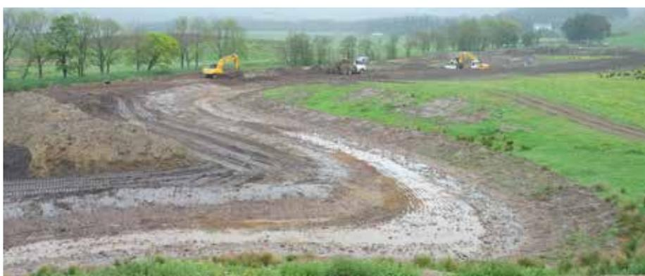
Figure 6.12. Implementing realignment works on the South Esk, Angus (© M. Halliday).
