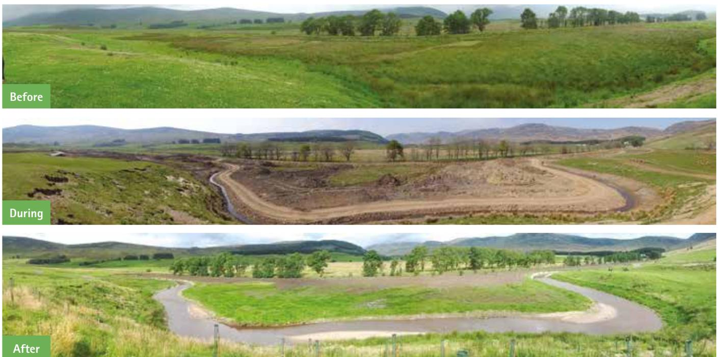
Figure 2.26. The Rottal Burn (South Esk), Angus, before, during and after work led by the Esks Rivers and Fisheries Trust to reintroduce meanders to a channelised reach: In addition to reducing flood peaks, this work sought to improve riparian and aquatic habitat and reduce the unnaturally high sediment load experienced downstream of the reach.
