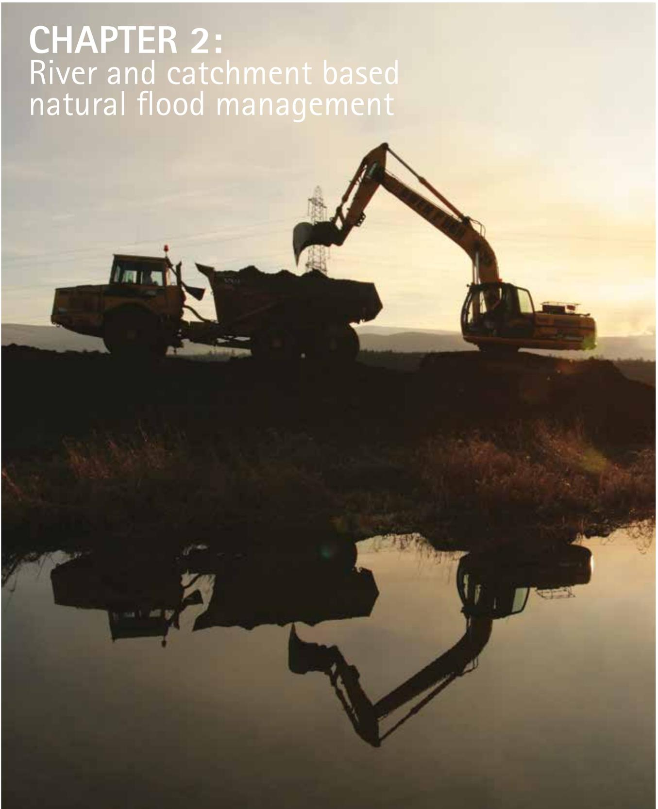
Figure 2.1. Removing flood embankments to provide greater floodplain storage on the River Till, Northumberland (© Tweed Forum).
