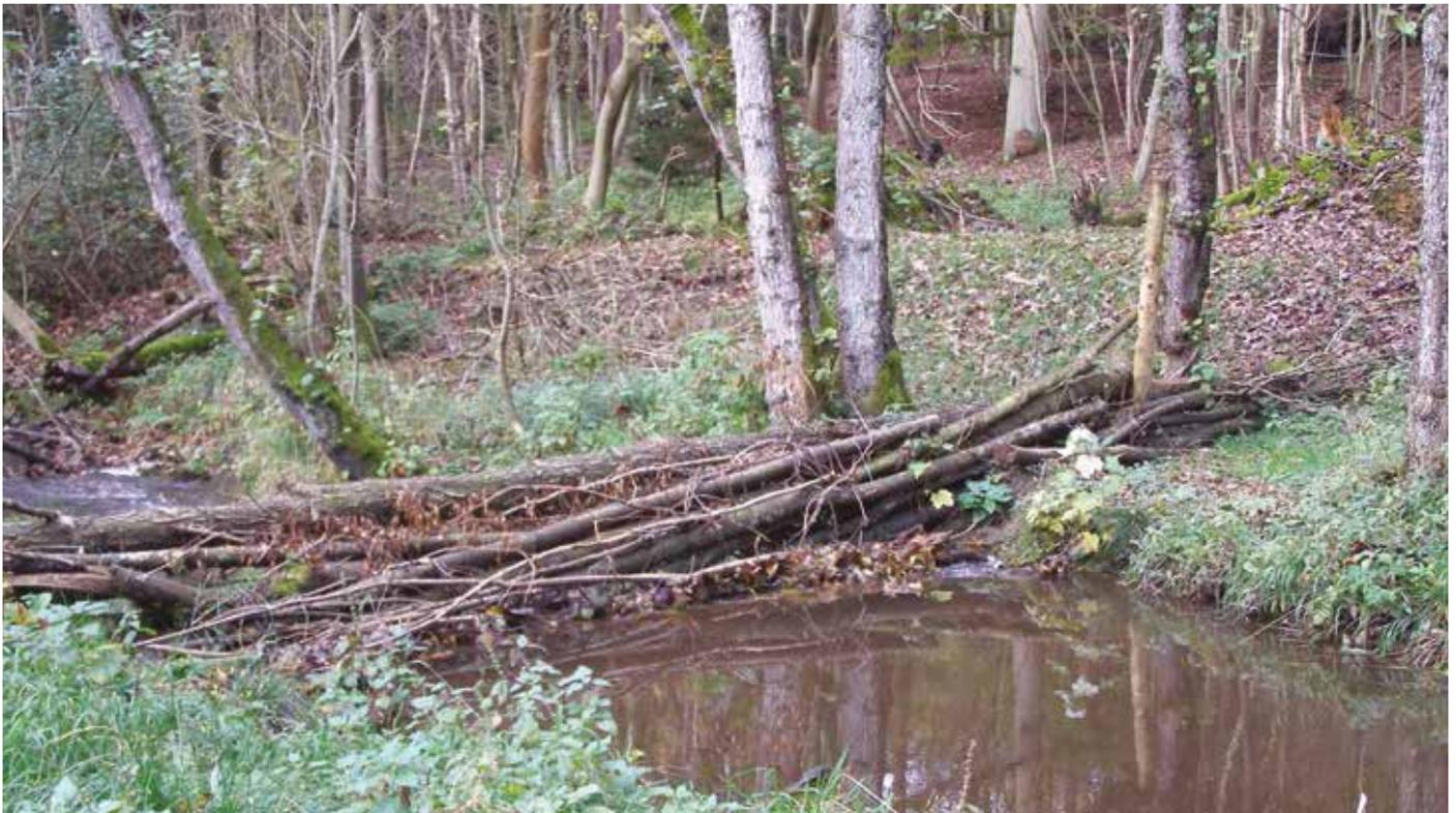
Figure 2.28. An instream structure, secured with a wooden stake, in the Pickering Beck catchment, North Yorkshire (©Forest Research).
